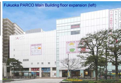
Fukuoka PARCO Main Building floor expansion (left)
