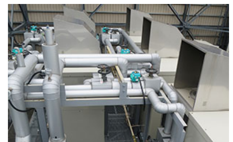
Grey water facility
