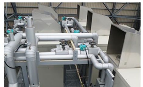
Grey water facility
